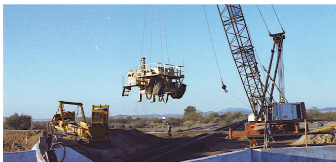
Trimmer is built in module fashion so components can be removed to reduce the weight of the trimmer and liner for lifting and transport in keeping with the available cranes and trailers available.
