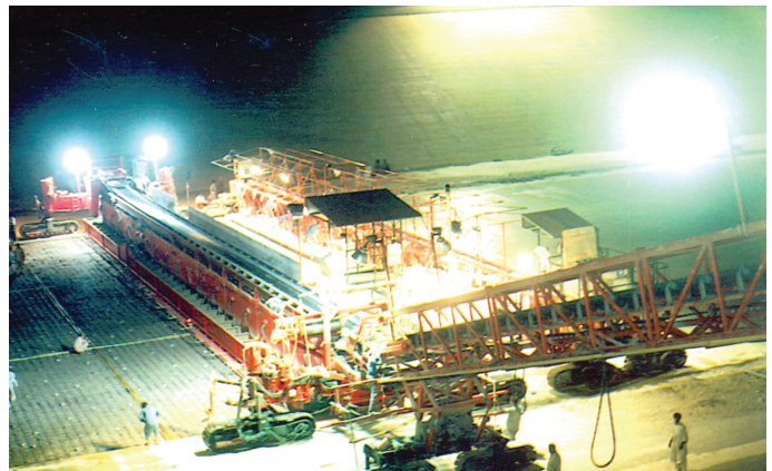
Self-propelled / self-moving auxiliary downhill feed conveyor to convey concrete into the canal bottom.
