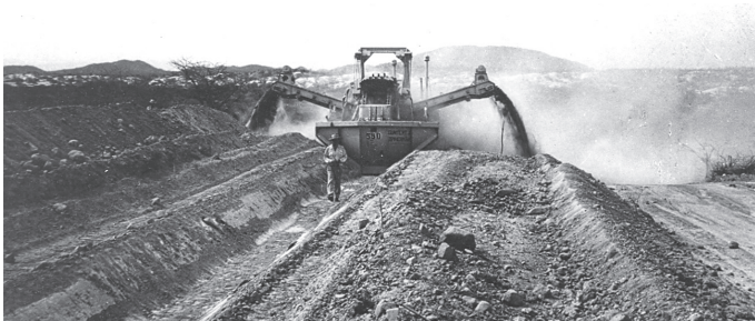
G&Z Canal Liner traveling on rails paving a canal bottom in Los Angeles, CA USA (1957).
