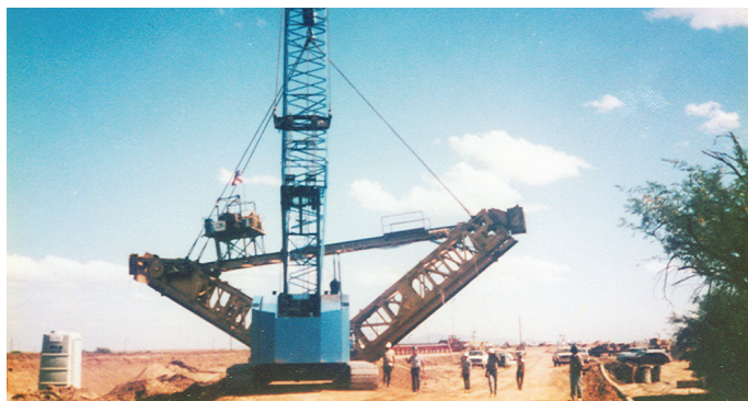
Full Span Trimmer being lifted by a 250T crawler track mounted crane around a structure.
