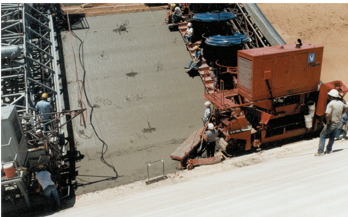
Automatic longitudinal joint inserters for inserting PVC cruciform shaped water stop (blue material on reels).
