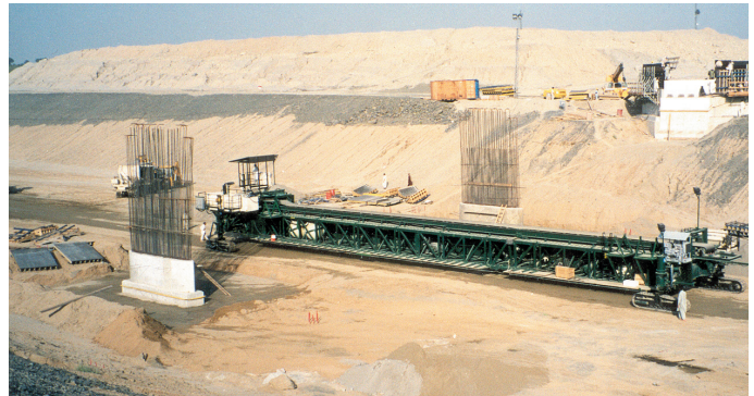
Half Span Liner in 90 degree steering mode walking and steering along the canal bottom passing a structure under construction.
