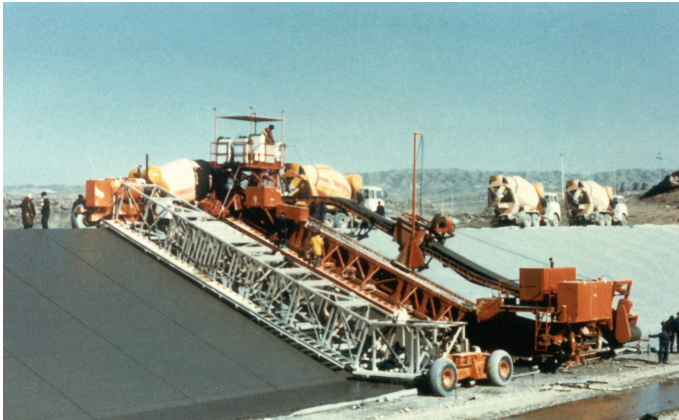
Two trucks discharge in a wiper conveyor.
