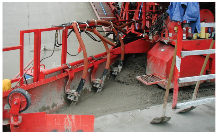
Back spreading device so bottom crawler track does not need to walk on the previously poured lining.
