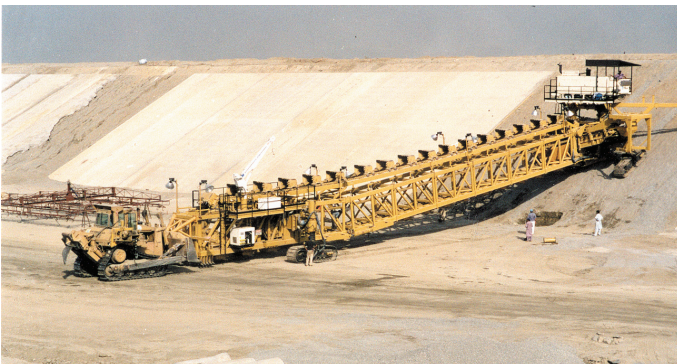
Half Span Trimmer walking up the slope under its own power if traction is available. In soft ground conditions a dozer may be required to assist.
