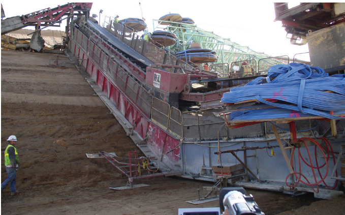
Subgrade guidance ski for elevation and steering control.
