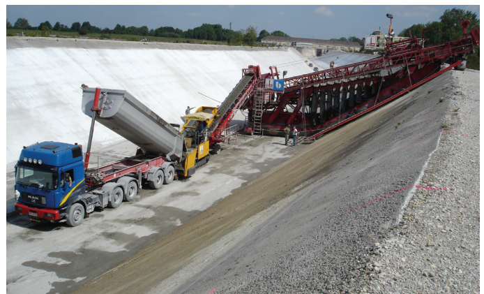
Semi-end Dump Trailer feeding a Concrete Placer.
