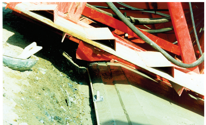
Hydraulically controlled curb forming module is available in any curb configuration needed.
