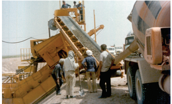
Single truck discharging into a concrete distributing car.
