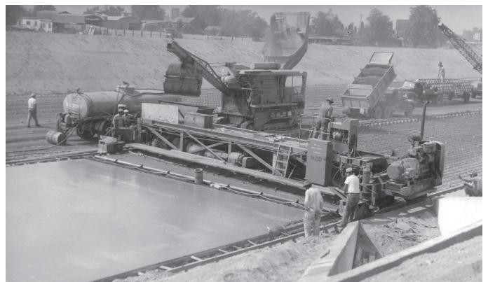
G&Z Canal Liner traveling on rails paving a canal bottom in Los Angeles, CA USA (1957).
