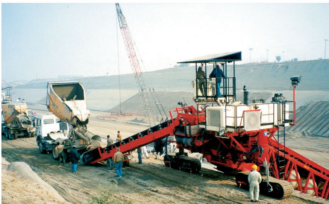
Agitator truck discharging into a charging conveyor.
